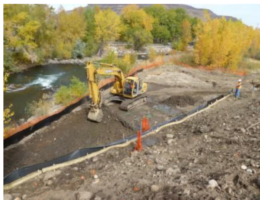
Radiological Technician oversees the removal of a 1-foot lift of contaminated soil. Prior to removal, a grid was established, and field screening instruments were used to identify areas requiring excavation.
